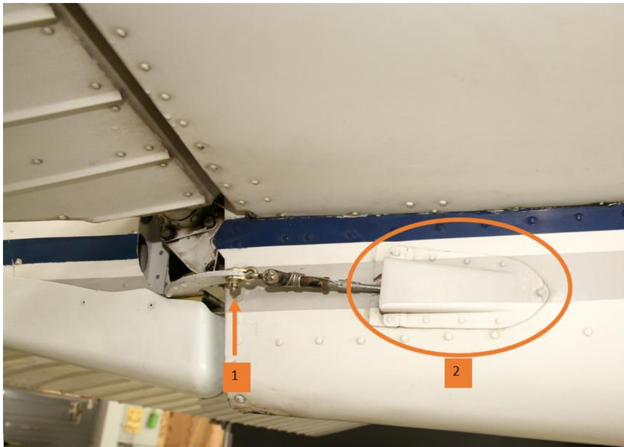
Figure 3-4, Tailcone Faring Removed and Rudder Cable
