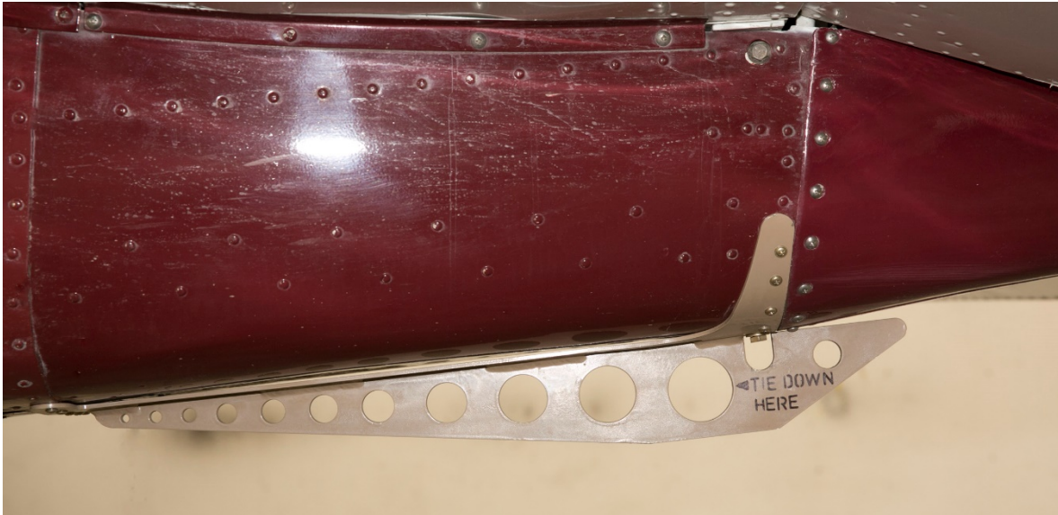
Figure 1-1, Replacement Tail Tie-down Installation
